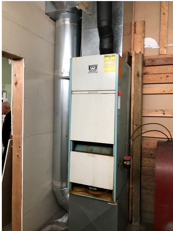
Photograph 4: Arena Interior – Oil Furnace
